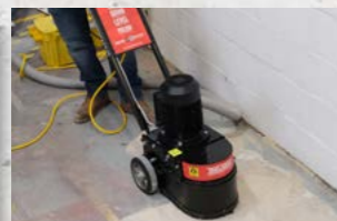
Grinding Concrete
