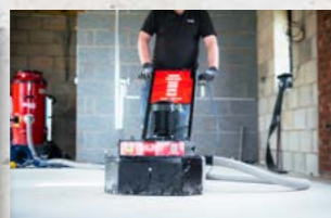
Removing High Spots
