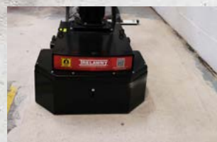
Polishing Concrete Floors
