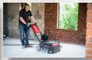
Grinding Concrete
